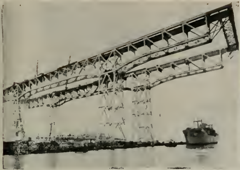
World's largest overhead traveling crane being erected in the San Francisco Naval Shipyard at Hunter's Point.
